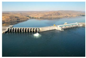
this reduced the crack opening width. A subsequent investigation showed that the primary cause of the fracture in the dam's spillway was a mathematical error made in the pre-construction design.
